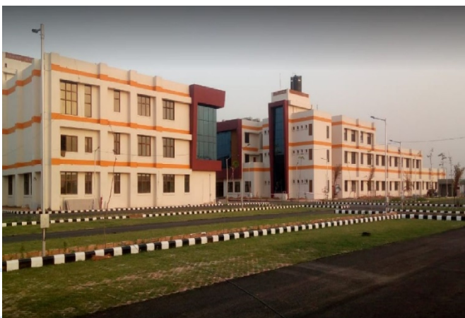
Newly constructed, MSME – TC Bhiwadi
